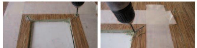
■ Using the power drill with the 2 mm (1/8") bit, drill continuous holes at a diagonal line from the outside corner of the plank to be replaced to the inside of the center piece that has been removed. Use caution not to damage the surface of the adjoining board or the foam underlayment.
