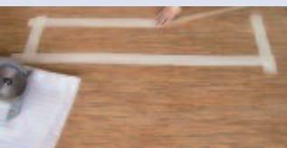
■ Apply masking tape around the board to identify the exact position of the plank to be removed and prevent exceeding the area to be cut. Mark the damaged plank approximately 2.5 to 4 cm (1-1.5") from the ends and sides.
