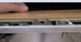
■ Set the circular saw blade to the thickness of the laminate plus 1 mm (1/32"). This will allow for easy removal of the plank. Use a left over board as gauge. If the foam underlayment is damaged
